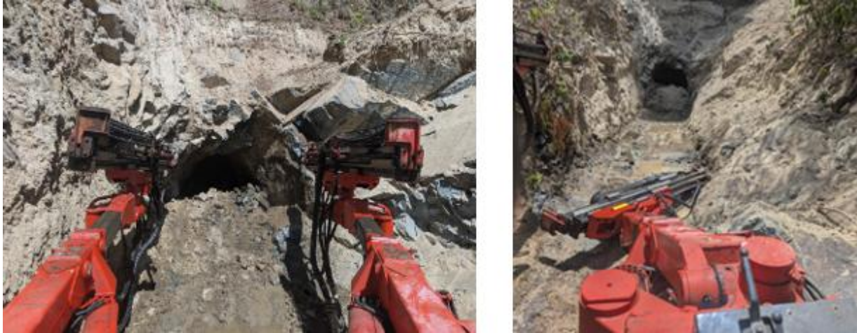
Figure 1 – Refurbishment of Dittmer portal entrance.
