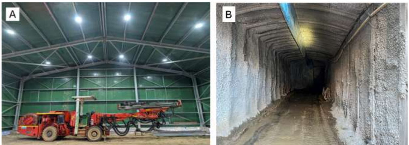
Figure 4 – Photos of the Dittmer mine development. (A) Completed acoustic shed; (B) Portal Shotcreting and Steel Supports.
