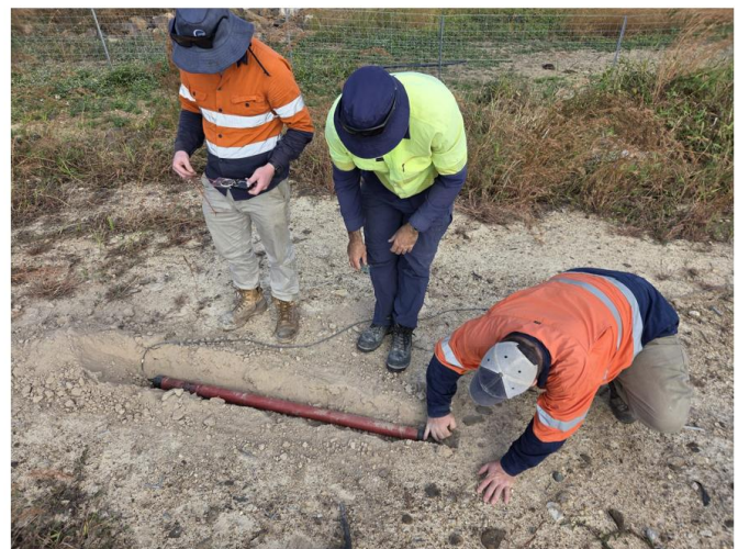
Figure 2 - Zonge field crew digging in sensors for the Dittmer MT survey.
