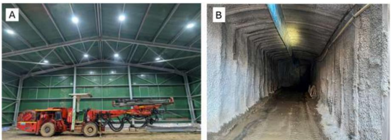
Figure 1 – Photos of the Dittmer mine development. (A) Completed acoustic shed; (B) Portal Shotcreting and Steel Supports.
